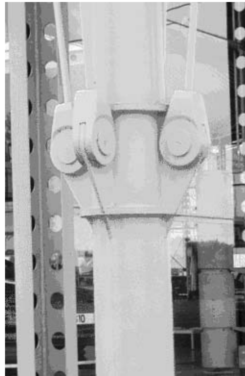
Renault Parts Headquarters Swindon – UK. Cast Connec- tion Details.
