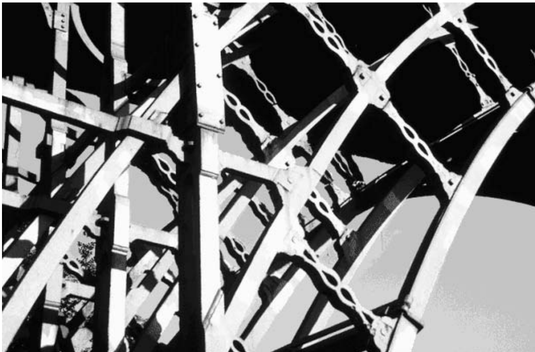
Details of World's First Cast Iron Bridge over the Severn. Built by Abraham Darby 1776–1779 at Ironbridge, Wales
