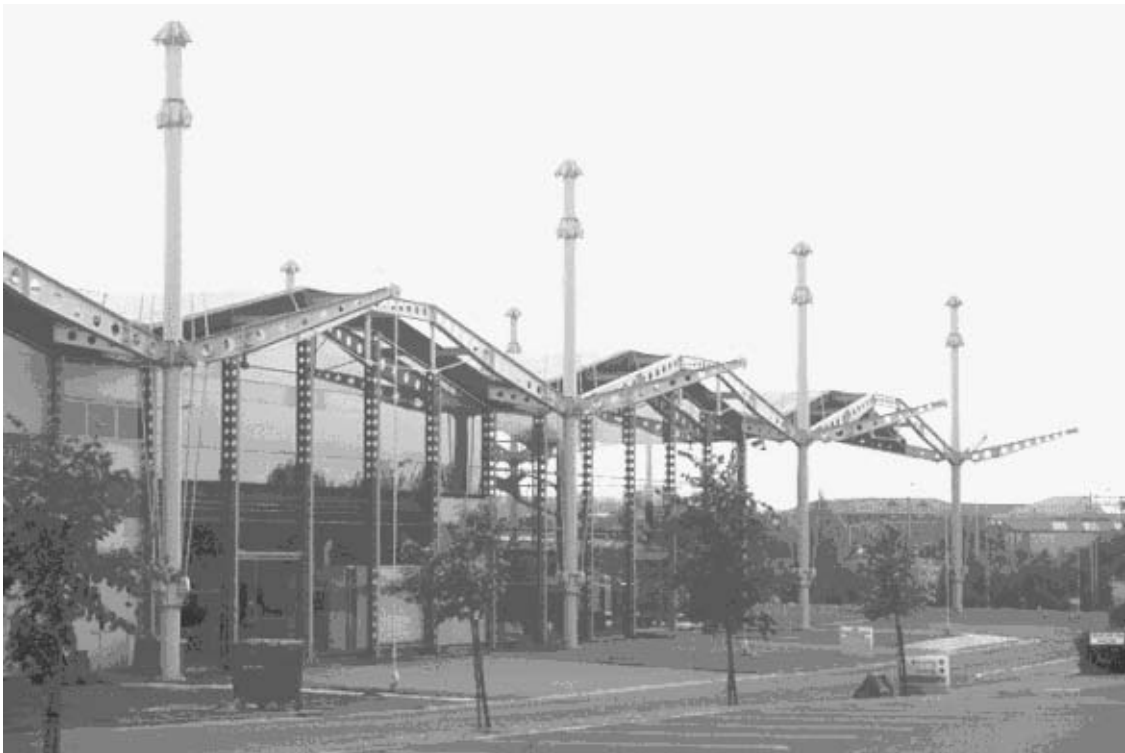
General Exterior View of the Renault Headquarters – Cable (rod) supported roof.
