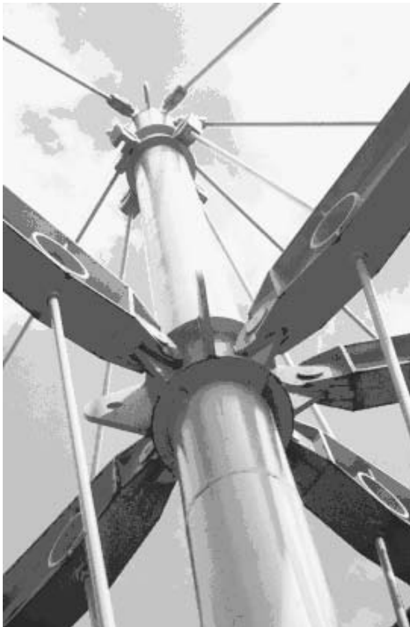
General Exterior View of the Renault Headquarters – Cable (rod) supported roof.
