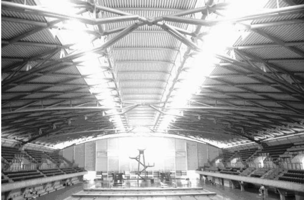
Ponds Forge Swimming Pool, Sheffield, UK. Cast Joints at arch hinges and bases
