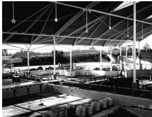
18 The bow string girder in position gives an overall lightweight look to the roof.
