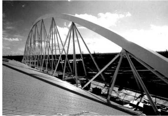
25 The design of the Aquatic Centre roof structure was required to be one which is capable of future expansion to Olympic mode in the year 2000. The Olympic mode requires a clear span structure of 138.6m to support the entire roof along one side as columns are not permitted in the viewing area. A structurally efficient arch was constructed for this using a light truss to prevent "snap through" buckling and provide the necessary flexural stiffness for non-symmetrical loads. The diagonal members of this truss are 19m long and are braced using a light cable system at approximately mid height to reduce the buckling length of individual members.
