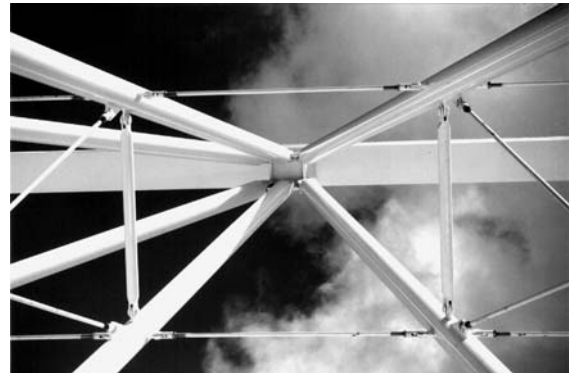
26 View looking up at Olympic Transfer Arch showing cable bracing of truss web members.
