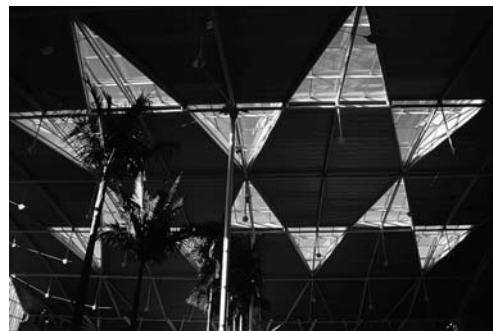
18 The bow string girder in position gives an overall lightweight look to the roof.
