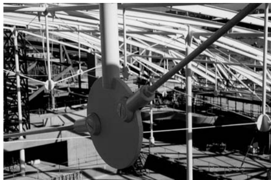
20 Bow string girder rods connected to vertical compression members using "off the shelf" forkends.
