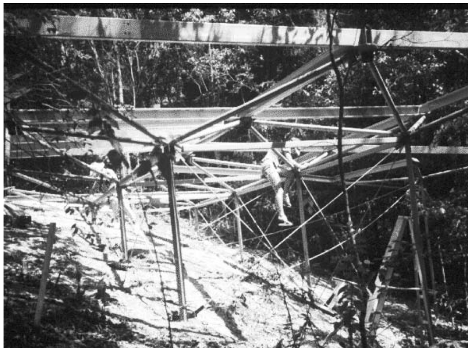
1st Quadropod House – Noosa Valley House
