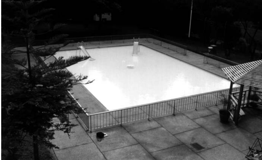
Figure 1. The wading pool prior to the shade structure
