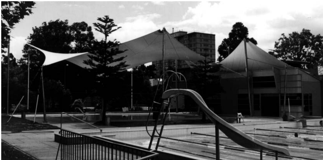
Figure 5. The finished shade structure, kiosk and entry.
