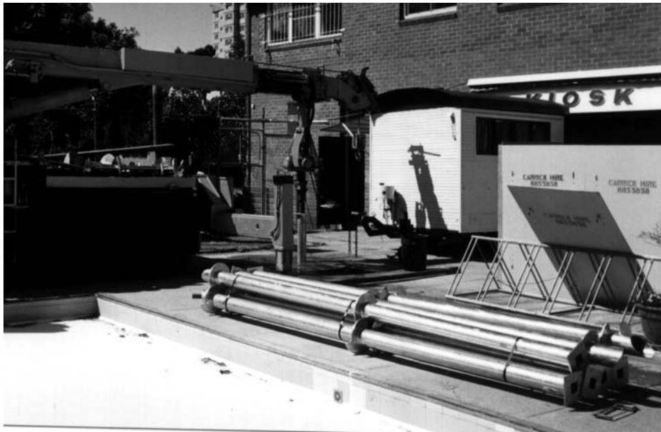
Figure 4. Compression anchors and installation equipment
