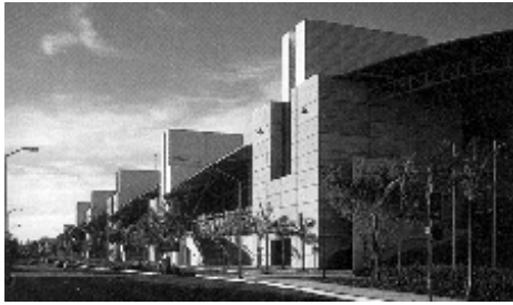
Left: From street level, the service towers clearly define the halls.
