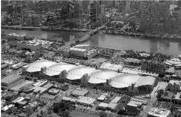
View towards north east with Brisbane River and city centre beyond. From right to left: principal elements are the main foyer, the Great Hall and Exhibition Halls 1–4. In front is the concourse, with the loading dock behind halls 2, 3, and 4. To the right of the loading dock is the railway plaza structure supporting the twin roofs of the ballroom behind hall 1 and the flat-roofed main meeting room and pre-function terrace behind the Great Hall. The complex occupies two city blocks with the dividing street passing under hall 2 and car parking on both sides under halls 1,3 and 4.
