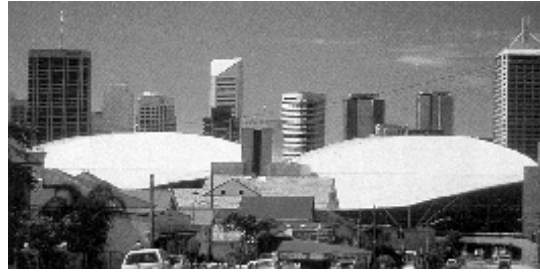
Right: From a distance the roof provides the principal visual impact
