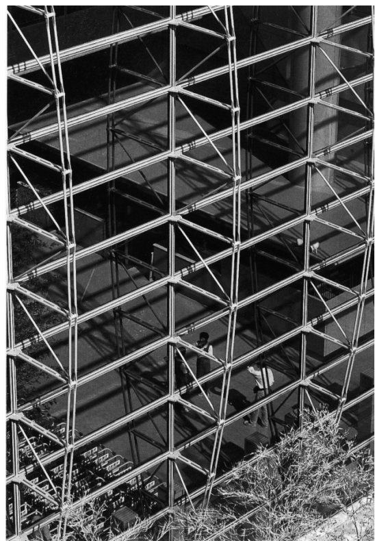
Figure No.4 View of framed glazing with bowstring trusses – Kansai Airport Source: Buchanan P (1994) Kansai, In The Architectural Review, No. 1173 Nov, 1994. p 78
