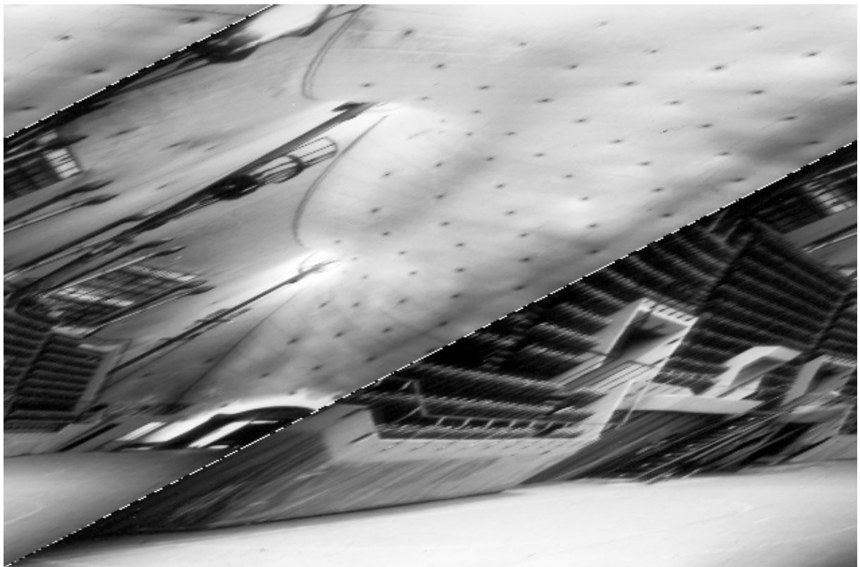
2.3 Double layer membrane with fibre insulating material
