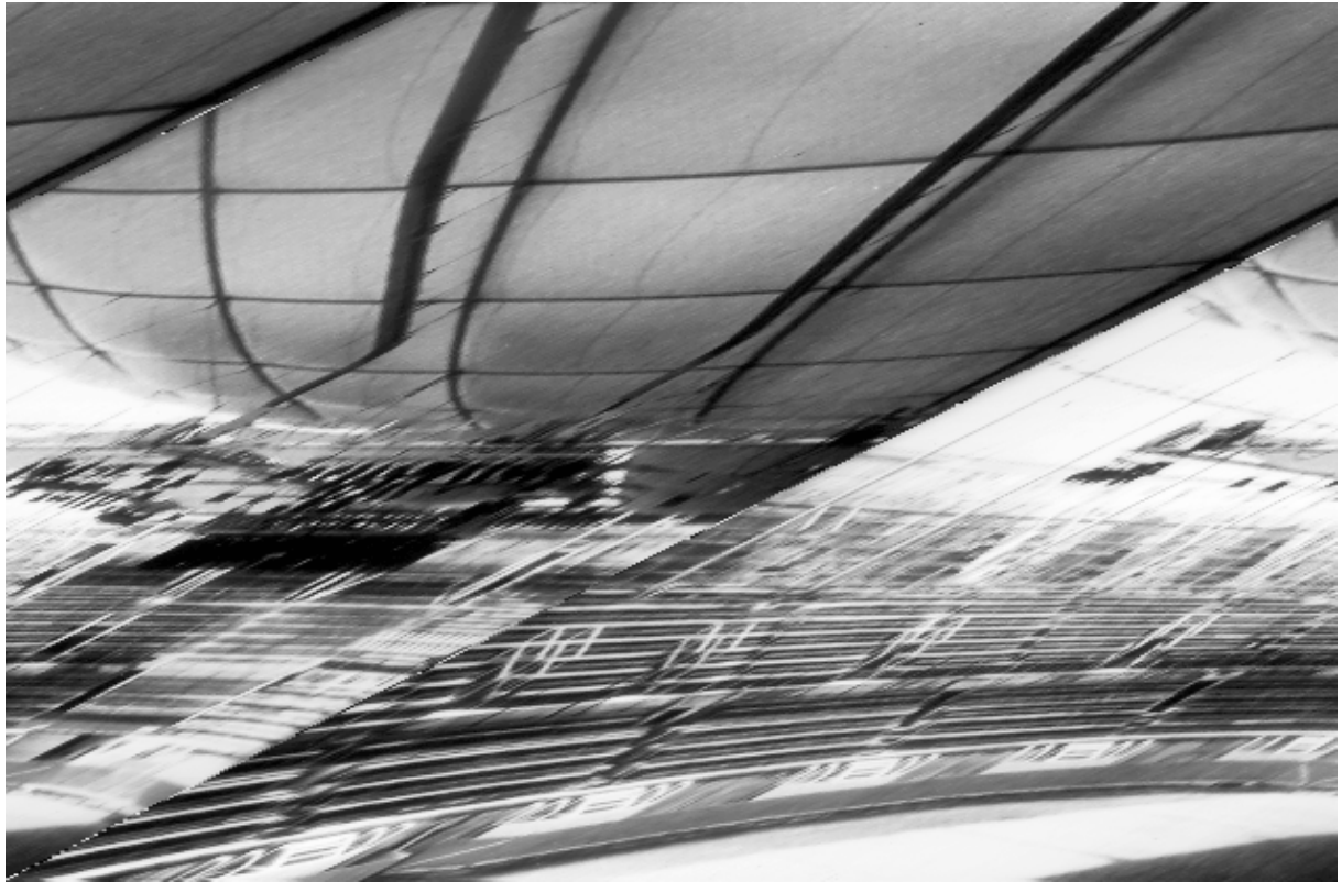
2.5 Double layer cushions with stationary air filling
