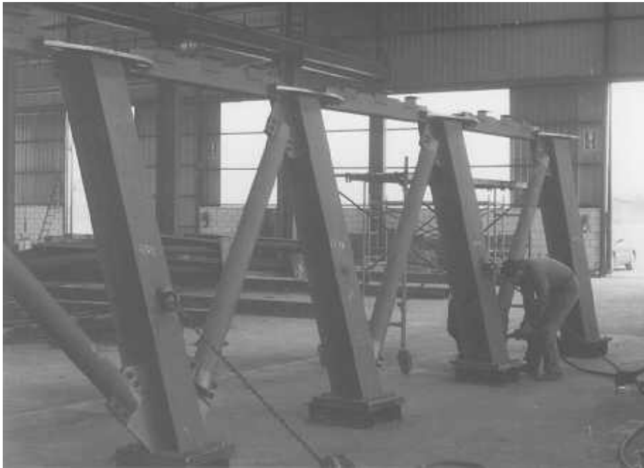
Figure 12 Horizontal Band Truss Shop Fabrication
