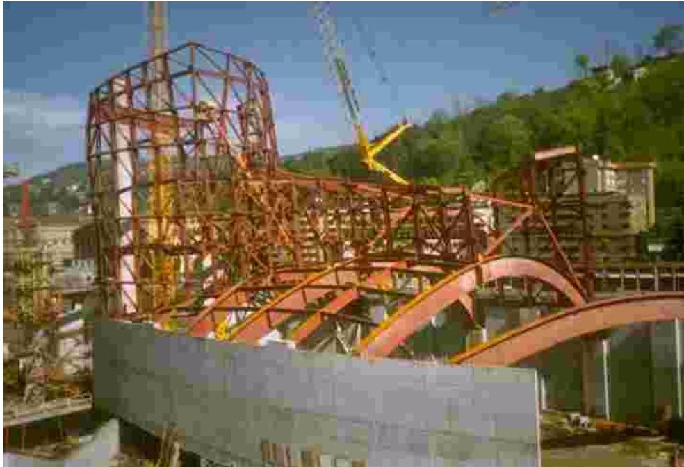
Figure 13 Boat Gallery - Under Construction
