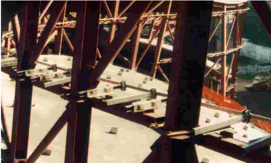
Figure 11 Secondary Structure Installation
