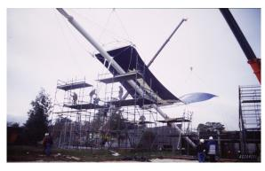
house non-linear structural analysis programme (FABLON). A number of full structural models were employed to assess the effects of various stay cable positions and prestress levels. Other runs were made to determine and assess the stability and cable load effects for various lifting positions during the erection sequence. The lifting points and phasing of the erection was critically analysed to ensure that the components were not subject to significant over stress or
