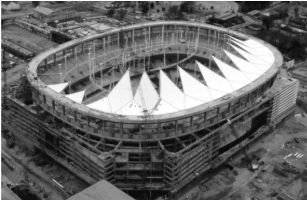
Figure 3. Georgia Dome during fabric installation
