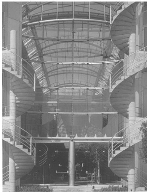
Figure 2 YKB view of glazed end wall
