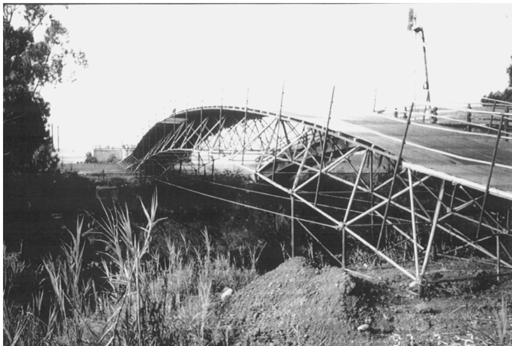
Figure 4: The constructed bridge viewed from the north bank
