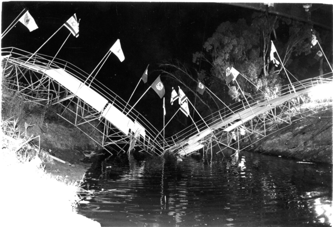
Figure 6: The collapsed bridge (Photo – Oren Agmon)
