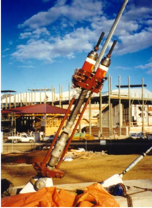
Tensioning Tie Down Cable
