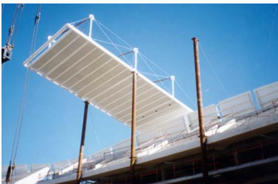
Erection of first roof panel
