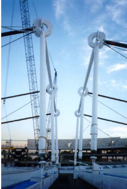
Roof panels being assembled on the ground.
