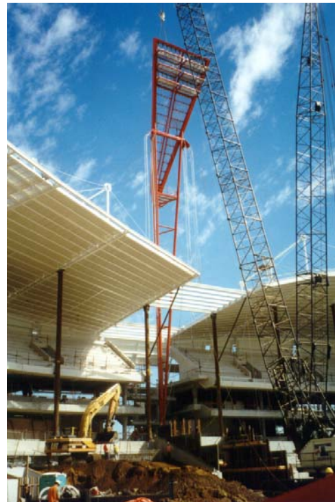
Mast Erection
