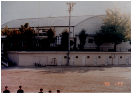
(a) Before collapse
