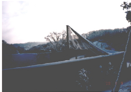
(b) Broken nets and a main pole
