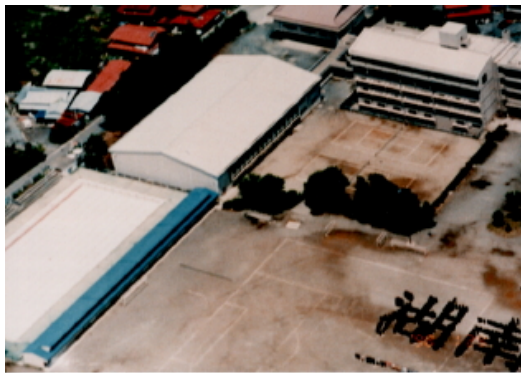
(a) Before collapse
