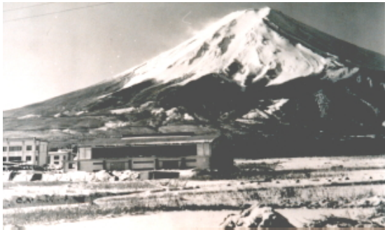
(a) Before collapse
