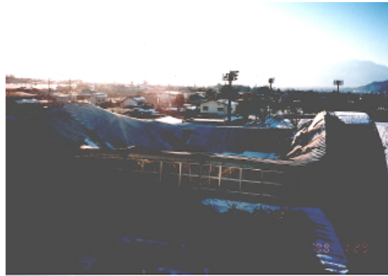
(b) After collapse
