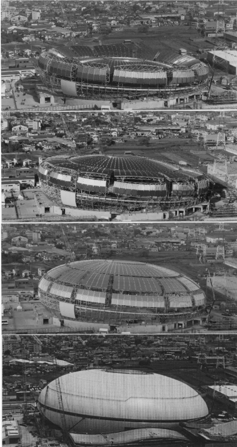
Fig. 4. Erection of “Namihaya Dome” by Pantadome System
