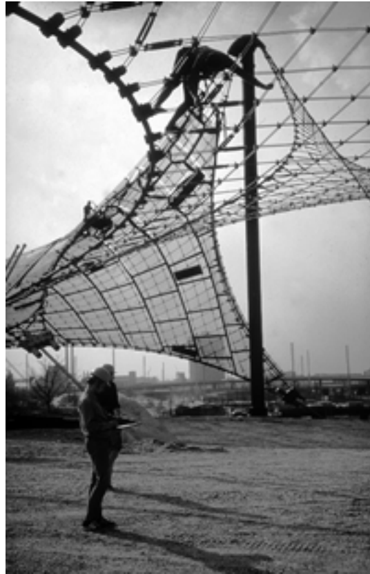
Figure 1: Munich Olympic stadium roof during construction.
