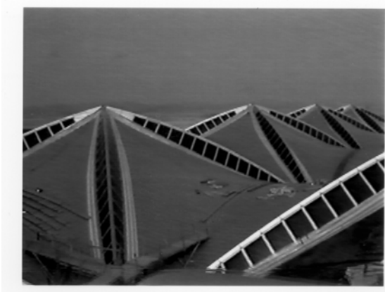
Figure 11 HP roof shell, (view to South)
