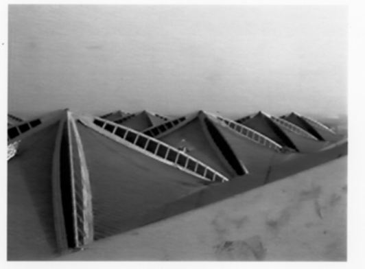
Figure 12 HP roof shell, (view to North)
