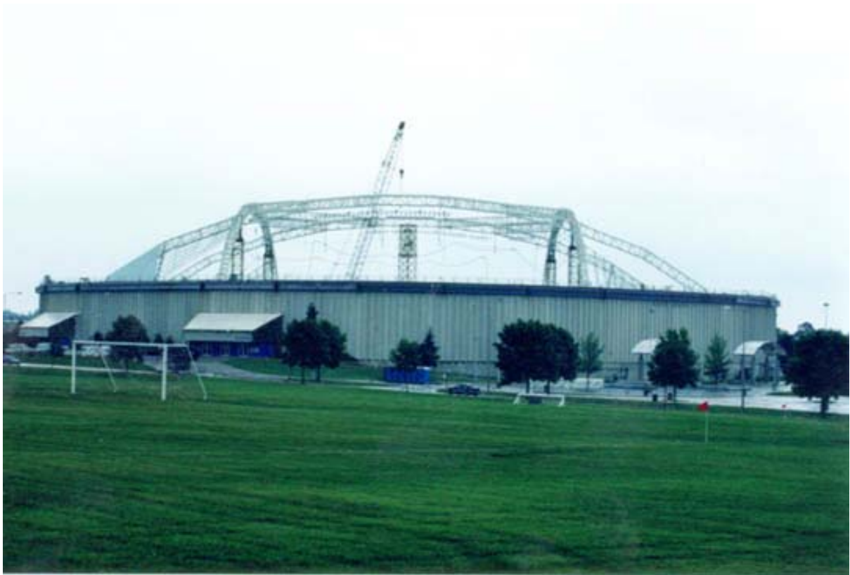
Figure 6 – UNI-Dome, Under Construction 6/18/98
