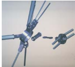
Fig.16 Detail of pre-stretching of hoop cable
