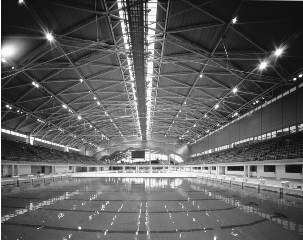
Figure 2. Lattice Shell Roof of the Sydney International Aquatic Centre (view towards North)
