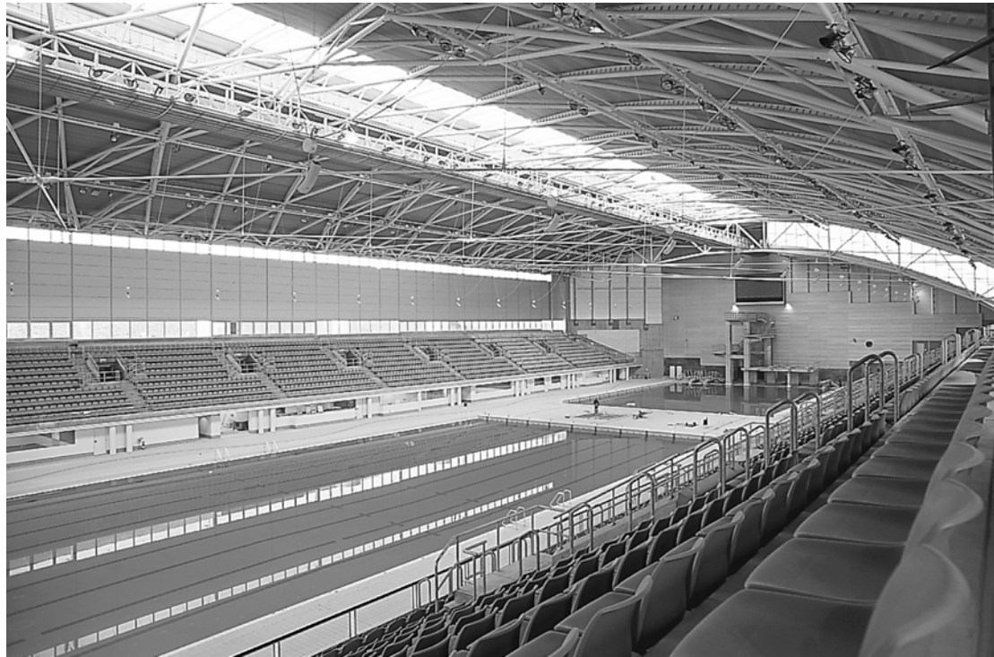
Figure 3. Lattice Shell Roof of Sydney International Aquatic Centre (view towards South-East)
