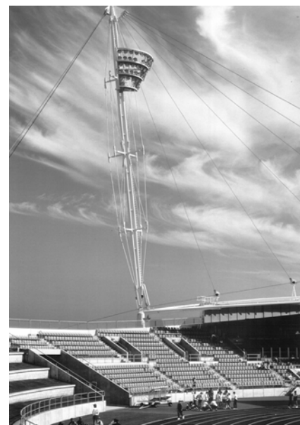
Figure 3. Cable-Stayed Multiple-Tube Mast
