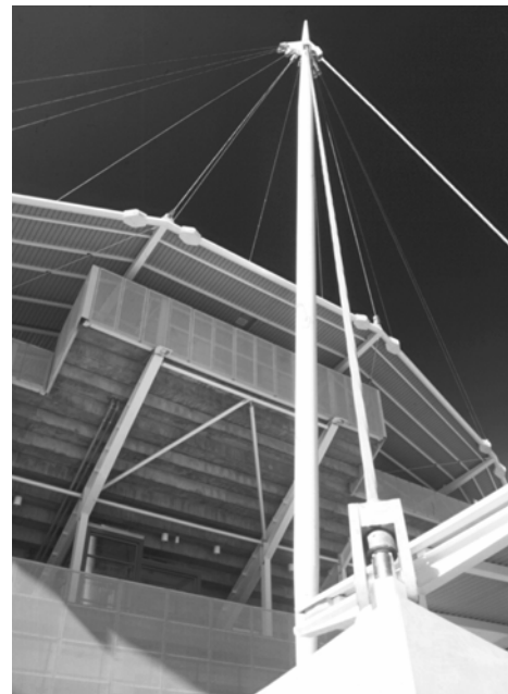
Figure 6. Mast Tied by Backstays
