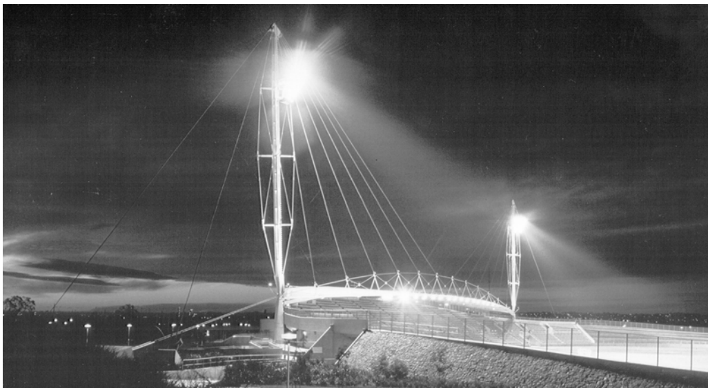
Figure 1. Cable-Stayed Roof of Sydney International Athletic Centre
