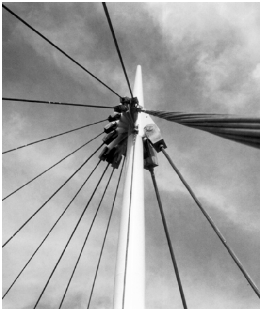
Figure 5. Stays Merging to Mast Head
