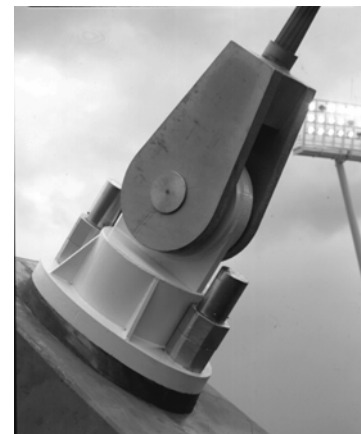
Figure 8. Uplift Load Resisting System
