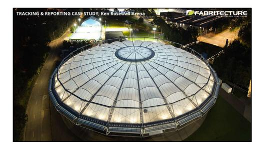
For our case study the Ken Rosewall Arena was been chosen. Its an innovative cable tensioned structure with PTFE fabric panels.
