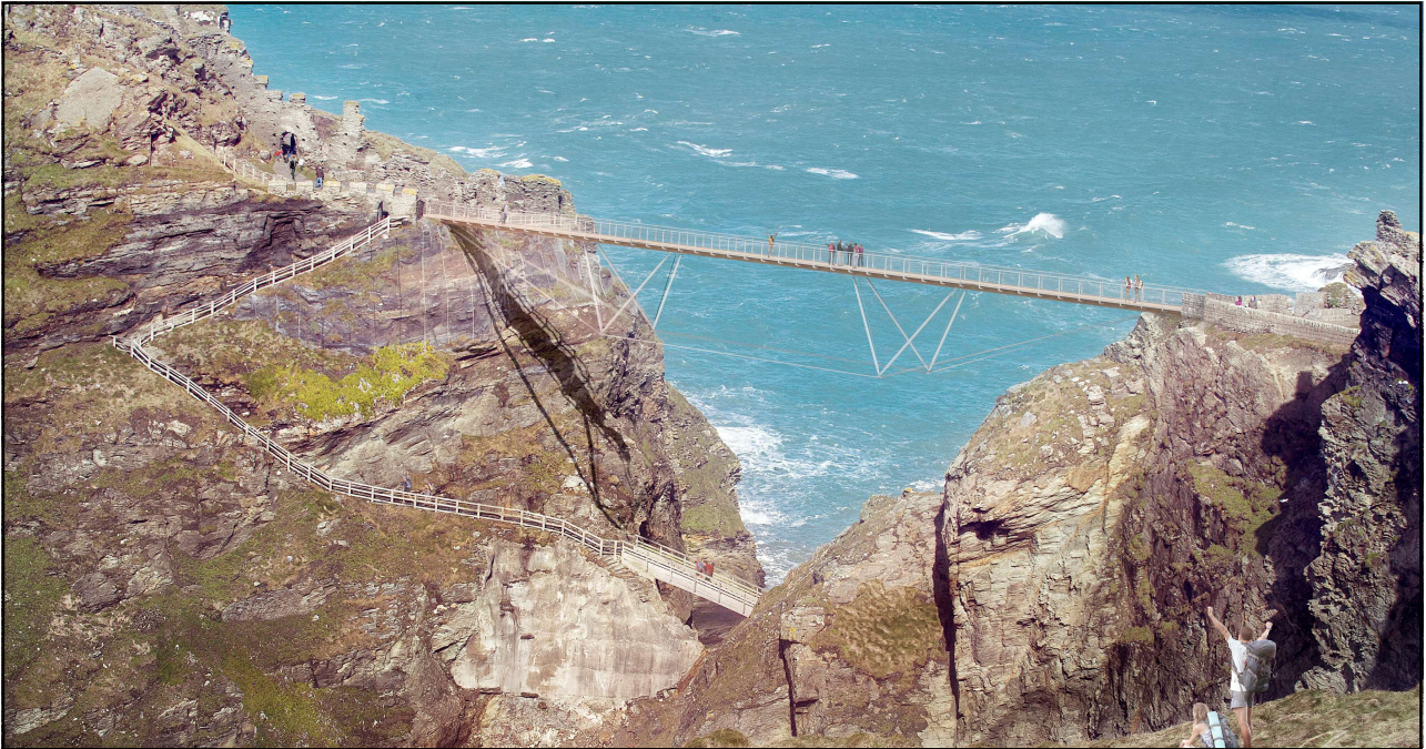
Lightness of structure – Tintagel Bridge, Cornwall
