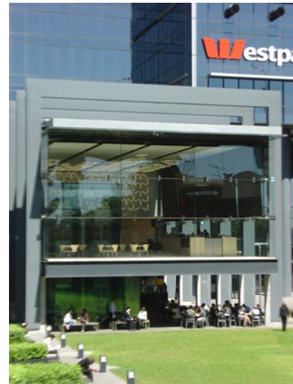
Figure 8 KENS Glass wall - glass with 14m horizontal tension cable
