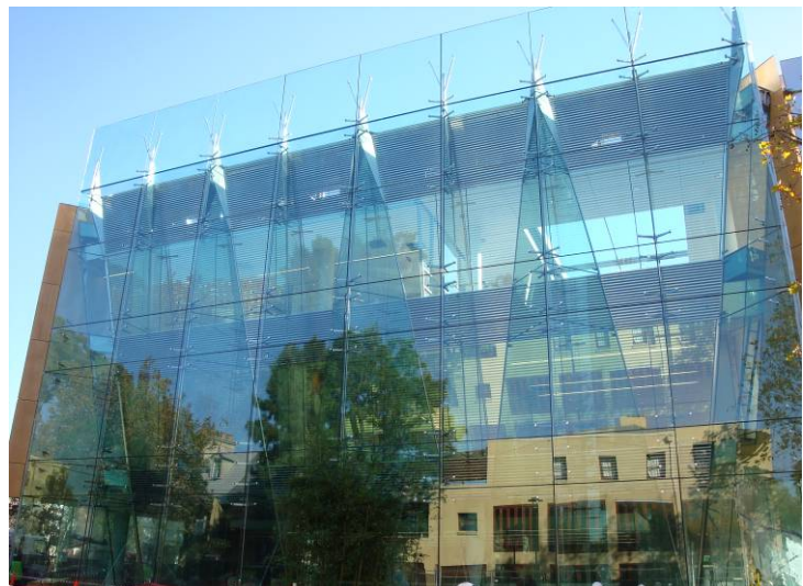
Figure 2 Surry Hills Library Structural Glass Wall
