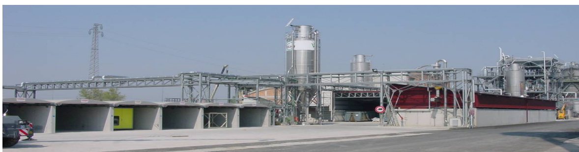
Full scale Industrialised Taxyloop Unit within the Vinyloop facility
