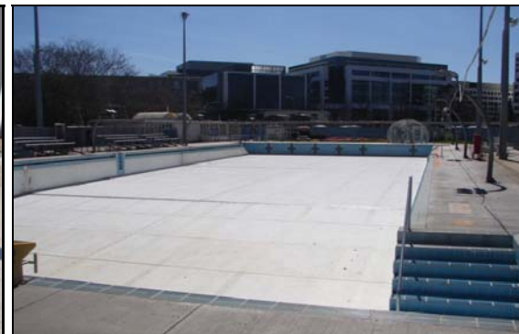
Cleared site ready in 2 days
