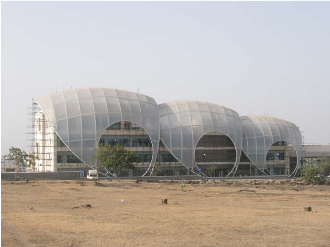
Figure 1. Fabric with 64% light transmission. Kirloskar Brothers HQ, Pune, India. (Photo courtesy of MakMax Australia)
