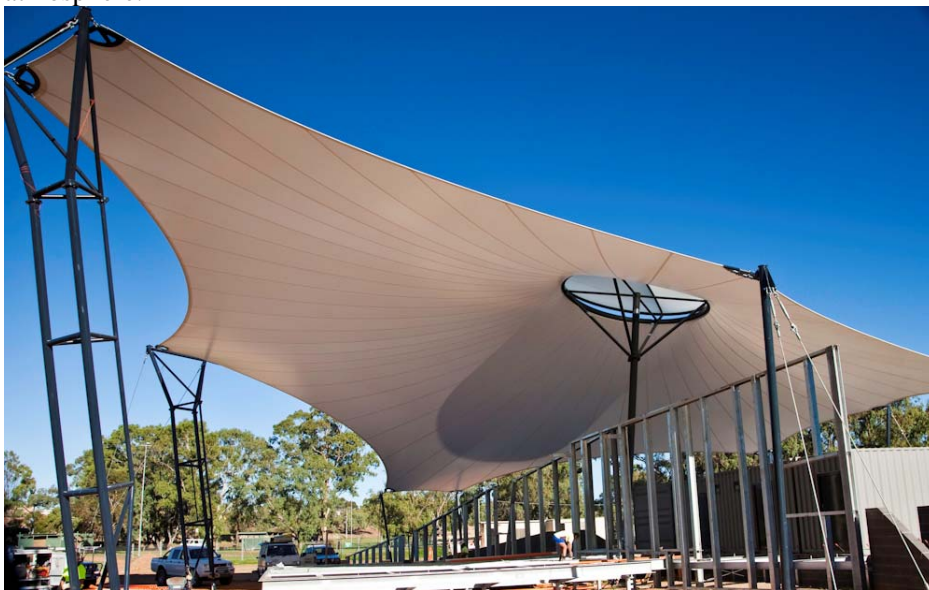
Figure 2. Semi-transparent fabric above central mast. Mildura Soundshell.
