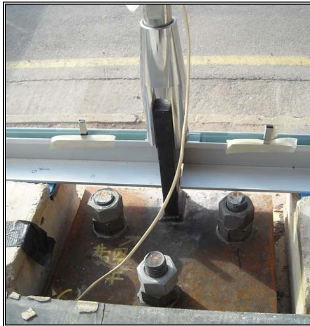
Figure 14: Photo of base connection during installation of the glass façade.
