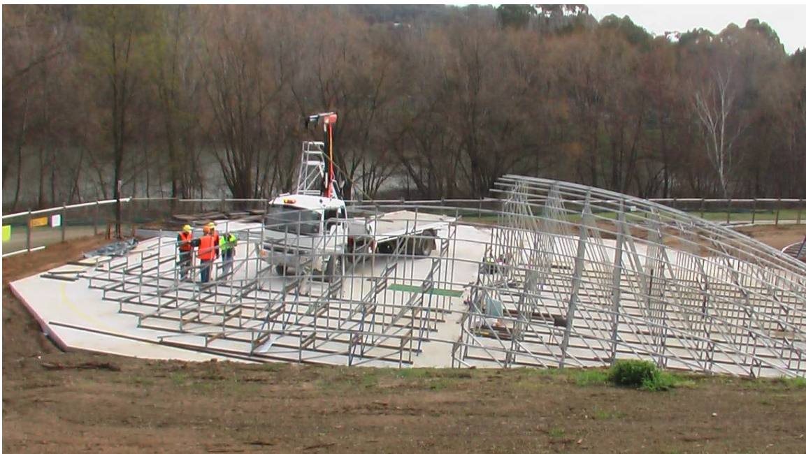
Fig. 2. Construction of the dish frame forming jig from a series of trusses.
