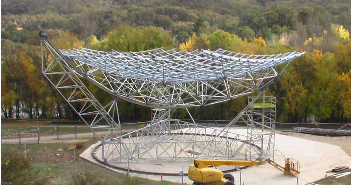
Fig. 6. Dish frame assembled on base-frame, with actuation systems in place.
