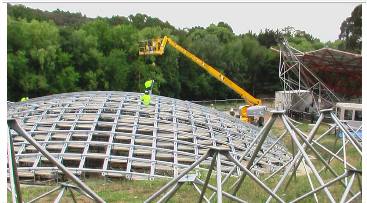
Fig. 3. Front surface of in-situ rolled sections joined in a square lattice by self piercing rivets. Prefabricated pyramid structural elements in the foreground.
