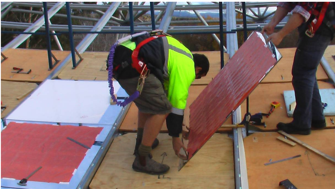
Fig. 7. Early stages of mirror installation on the dish surface.
