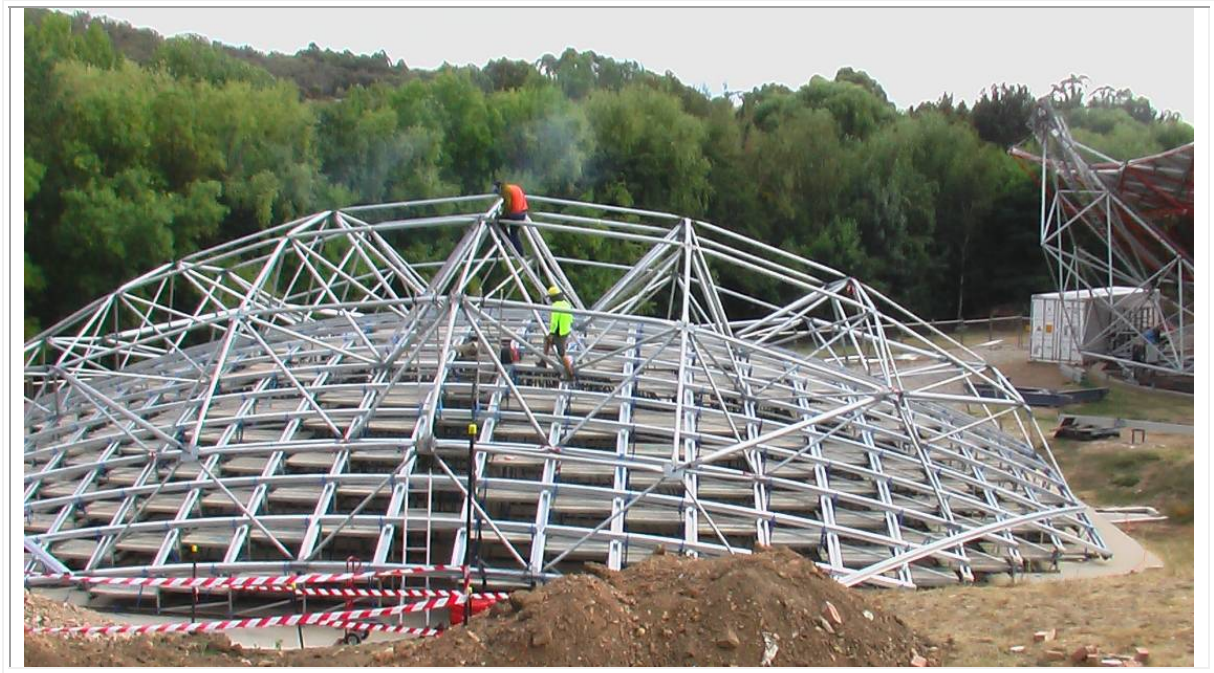
Fig. 4. Dish frame with pyramids installed and back surface chords being welded in place.
