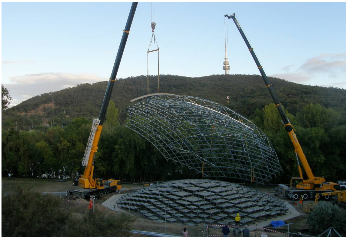
Fig. 5. Removal of the completed dish frame from the jig.
