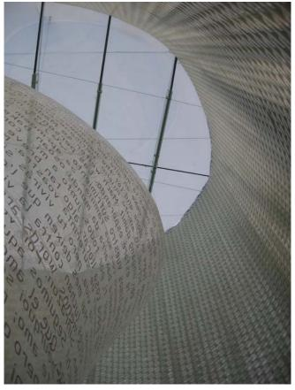
Converting this shape to cutting patterns for fabrication was further constrained by the requirements of printing. The seams themselves needed to be horizontal, with additional horizontal reference lines provided for the text itself.
