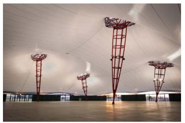
The structure demonstrates the integration of the need to design with "construction in mind". The end result is a very lightweight support steel structure (less than 10 kg per square metres) with clean and simple lines and form.
