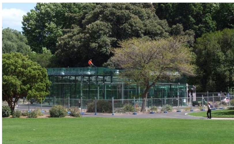
Figure 5 Construction Worker Cleaning Glass Roof – Viridian 'Activ' Coating will reduce the frequency by which this is required (photo Jeremy Prentice, DEH)
