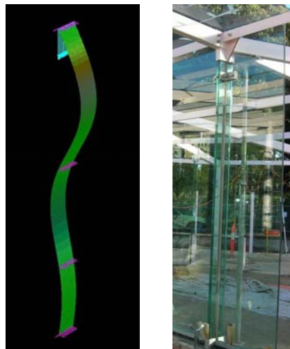
Figure 6 Glass Column - buckling analysis in Strand7 and final installed photograph
