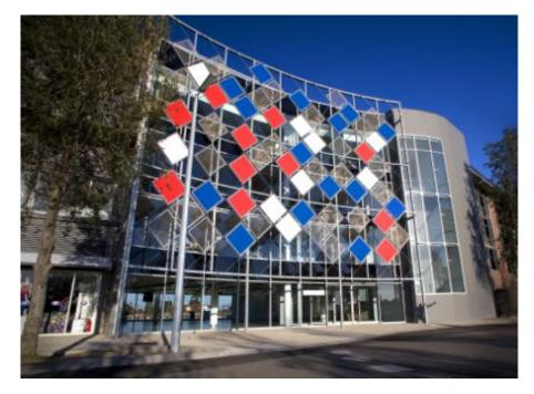
The Whitten solution with its cable grid of 8mm stainless cables and cross clamps is truly individual. Like most tensile structures in glass, metal panels, timber or tensioned fabric, the integrity of the lightweight solution relies upon geometry and pre-stress in the cables to reduce deflection and
