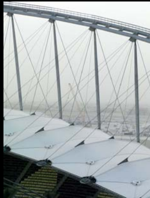
Khalifa Stadium, Doha, Qatar
