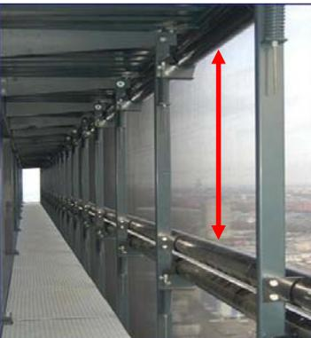
**Warp direction** (width of floor) fixed rigid with kedar system.
