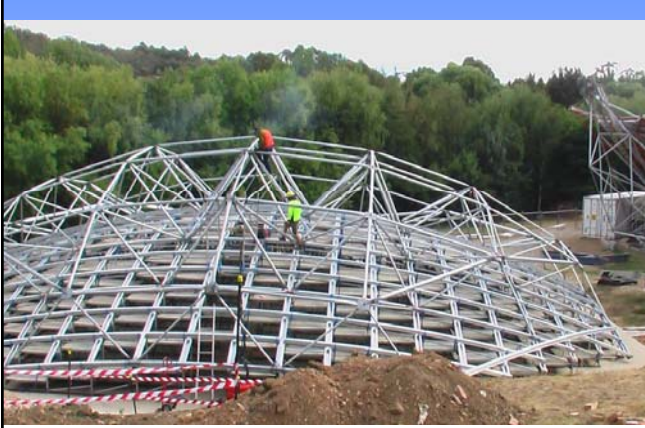
Welding of spaceframe
