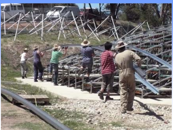
Installation of front surface members
