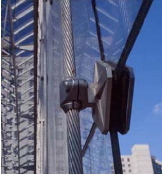
Figure 6 - Clamp Detail
