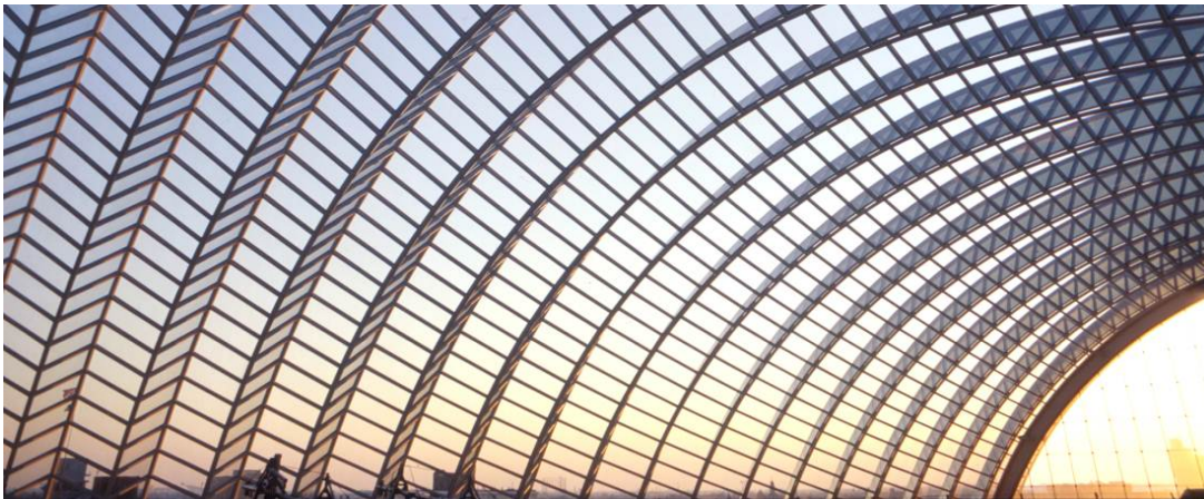
Figure 4a - view along roof to end wall
