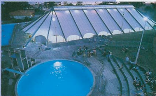
Gisborne Olympic Pool Cover Matrik Structures Pty Ltd
