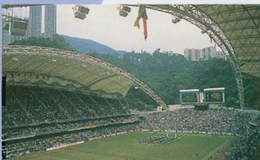
Hong Kong Stadium Roof Bond James Norrie Marsden Pty Ltd
