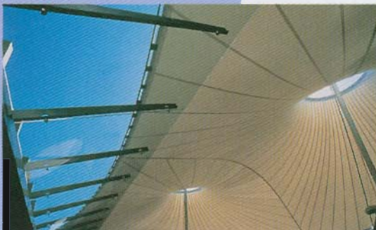
Porirua Covered Walkway Architects Workshop Ltd
