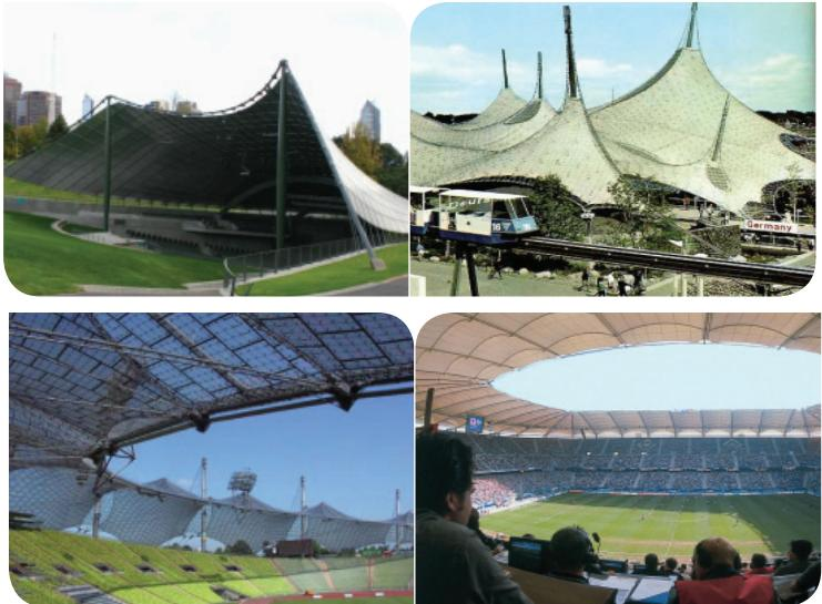
Frei Otto's German Pavilion at Expo 67 was the fore runner to his famous Munich Olympic Stadiums. Many large modern stadia have been built using a cable structure supporting, and giving form to tensioned fabric roof panels. With a complete stadium, the inner opening has a large tension ring made from cables. The radial cables are tensioned and resisted by an outer compression ring which in turn is supported by many outer columns. Connections and cable end fittings are a vital part of the design.
