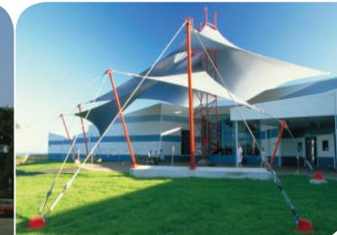
To obtain the curvatures, major support elements such as masts and arches are used. Fabric materials include teflon or silicon coated glass, PVC coated Polyesters, foils and shadecloth.
