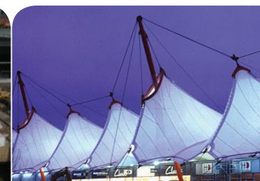
The main design loadings are the initial prestress in the fabric and wind loads - dead weight is very small. Prestress is generated by patterning the fabric from standard width rolls to be a smaller size. The fabric is stretched to its supporting system by adjusting the length of edge cables, tensioning of side guys, jacking up of internal masts or a combination of methods.
