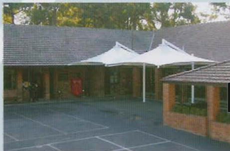
All-weather ambulance canopies, transformed an outdoor covered area for a school.
