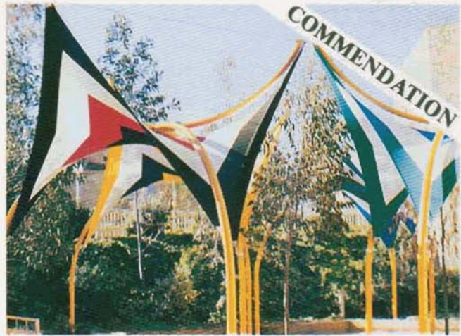
TENSILE STRUCTURES, PERTH, W.A. SHADE PODS, CULTURE CENTRE, PERTH.
