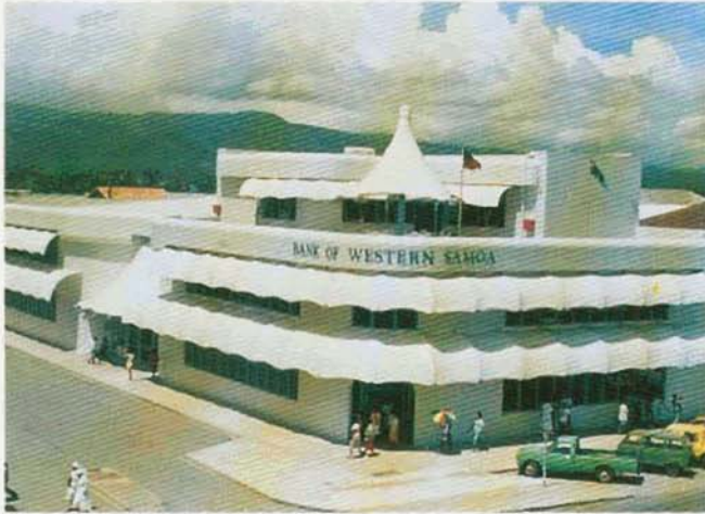
STRUCTURFLEX, AUCKLAND, N.Z. BANK OF WESTERN SAMOA.
