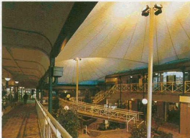
COVERTEX (AUST.) PTY. LTD., BRISBANE, QLD. 'MAYFAIR ON THE BAY' SHOPPING CENTRE, HOBART, TAS.
