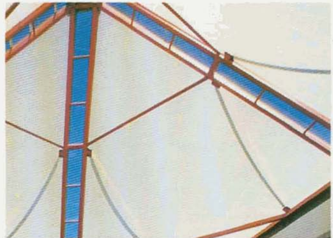
TENSILE STRUCTURES, PERTH, W.A. THE LIGHTHOUSE RESORT.
