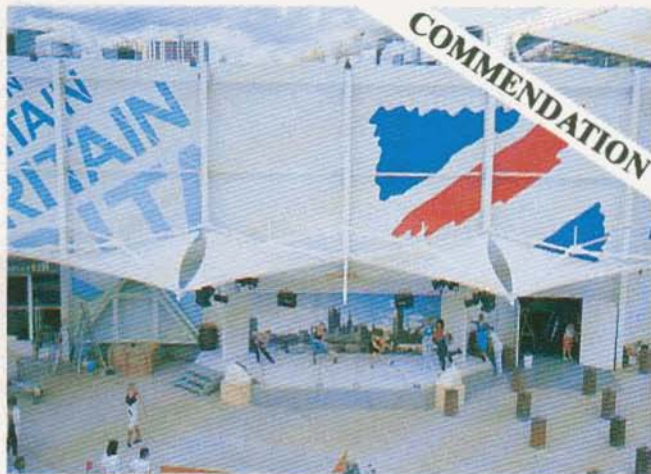
SHADE STRUCTURES PTY. LTD. (QLD.) STAGE ROOF, U.K. PAVILION, EXPO 88, BRISBANE.
