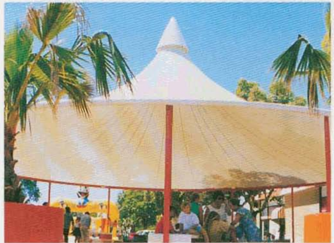
TENSILE STRUCTURES, PERTH, W.A. MIDLANDS GATE SHOPPING CENTRE, PERTH, W.A.
