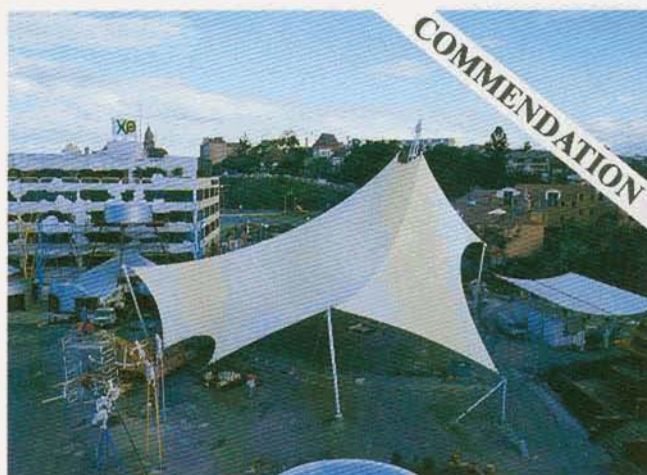
SPACETECH PTY. LTD., MELBOURNE, VIC. EXPO 88 GATEWAY STRUCTURE, BRISBANE.
