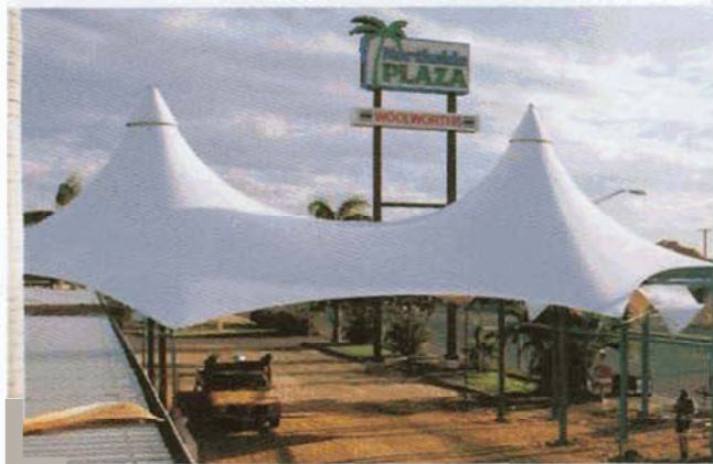
NORTHSIDE PLAZA ROCKHAMPTON Structureflex Australia
