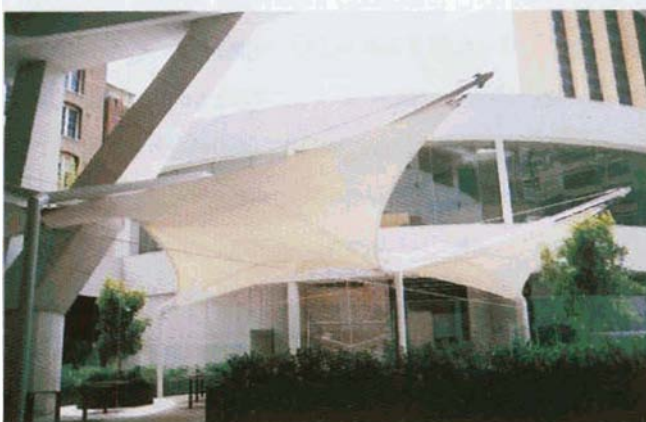
GROSVENOR PLACE COFFEE SHOP Kamol's Membrane Structures P/L
