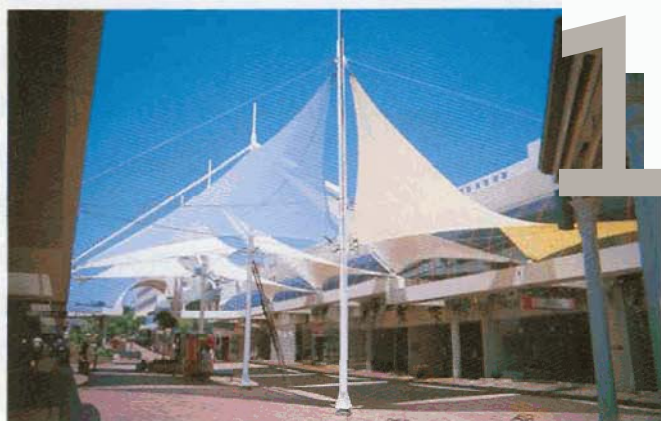
IPSWICH CITY MALL Kamol's Membrane Structures P/L
