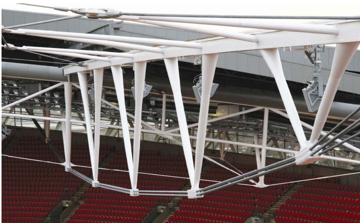
FIGURE 3: SEMI-VIERENDEEL RUNWAY TRUSS
